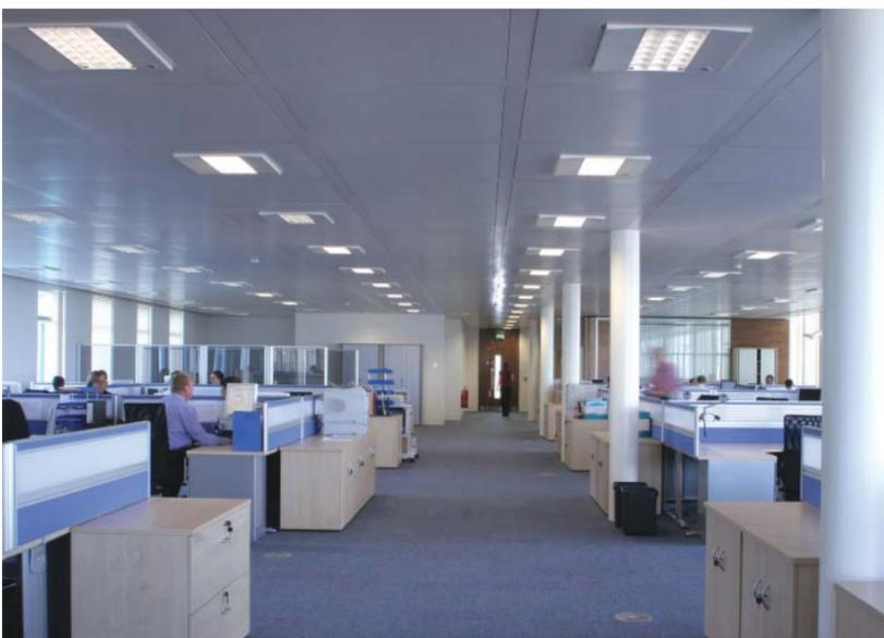
Chilled ceilings and beams use water as the cooling medium
